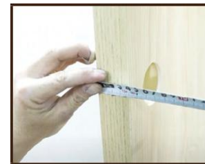
Step 12: Install lock set and accessories.
