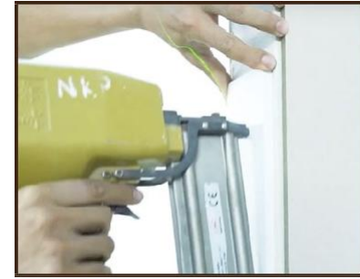
Step 3: Attach the pads into the wall with the laser ruler, make sure to attach the pads in a straight vertical line.
