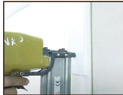
Step 4: Install the hinge side frame first.
