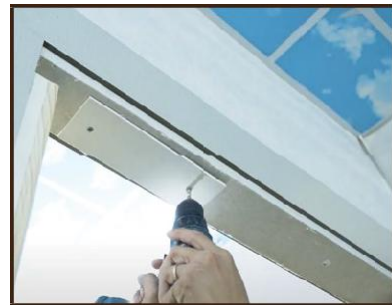
Step 8: Install the horizontal frame.
