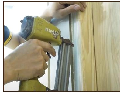
Step 7: Adjust and install the other vertical frame
