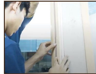
Step 9: Install the plastic seal to damp and soundproof.
